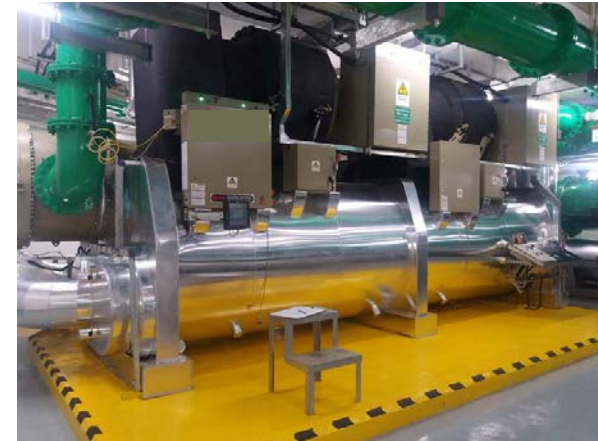
Chiller Replacement Completed
