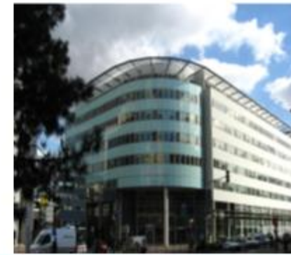
Office building, Lyon 17k m 2 , 165kWh/m 2 -a
