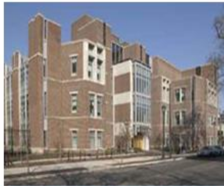
Office building A, USA 6425m 2 , 364kWh/m 2 -a
