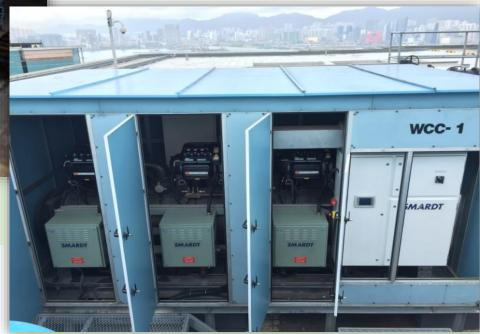
Enclosure for oil free centrifugal chiller
