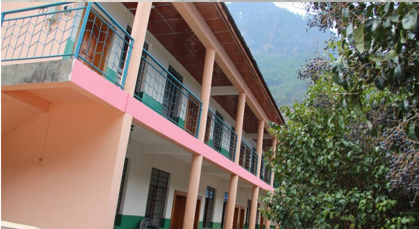
Vacant village primary school building
