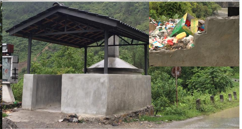
Rural garbage incinerator—Concerning rural pollution, but with weak maintenance and management
