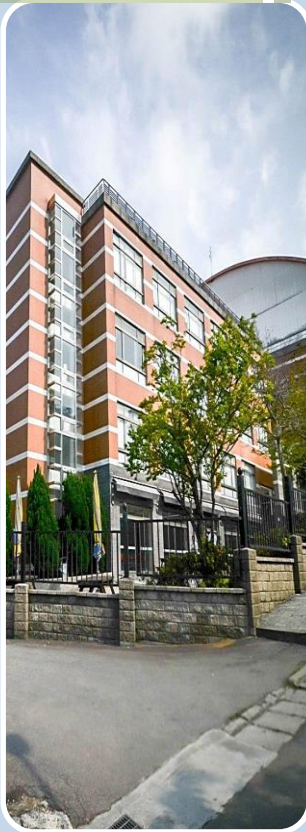
The public new buildings
