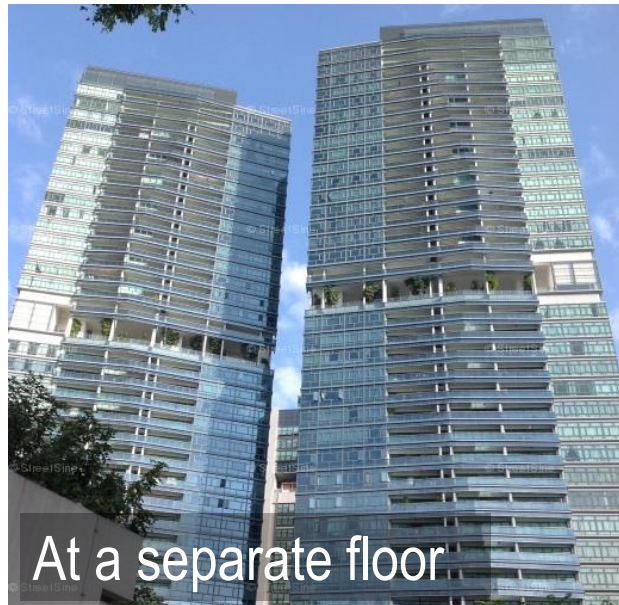
Connecting all towers
