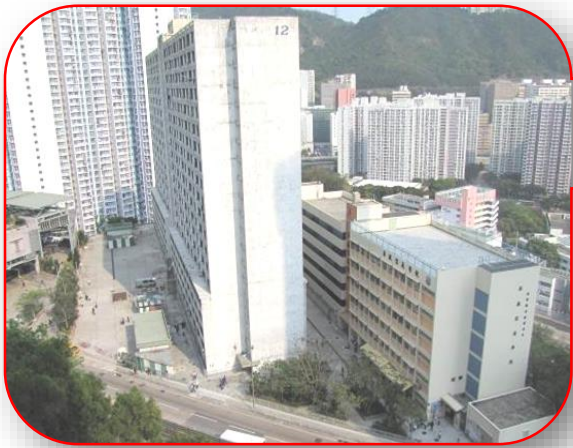
Former Block 12 and the existing school adjoining to the site.
