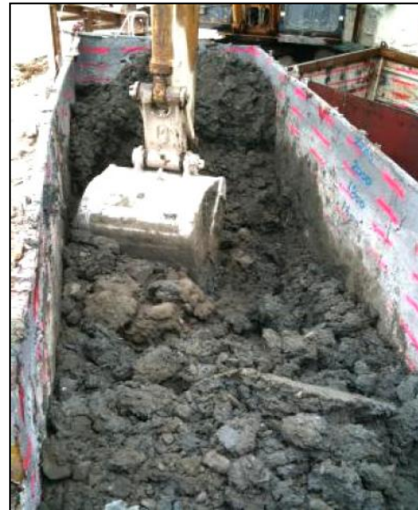
Mixing with cement and granular material
