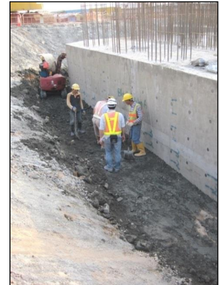
Backfilling with stabilised marine mud
