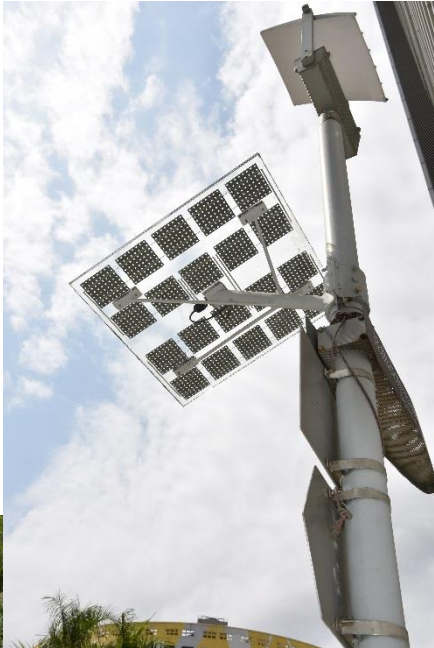
Solar powered lamp pole
