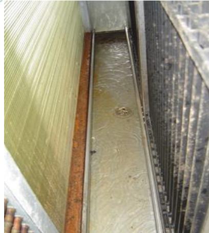
Recycle condensate water of AC system
