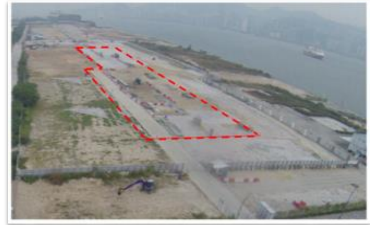
The South Plant located at underground of former-runway of Kai Tak Airport
