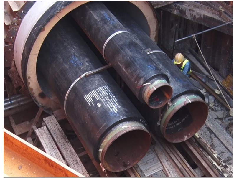
DCS Pipes Laying inside the Underground Tunnel
