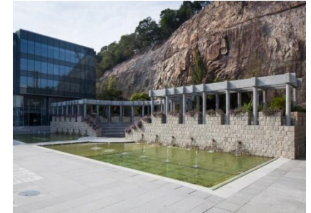
Mall Garden restored with Pools & Skylights
