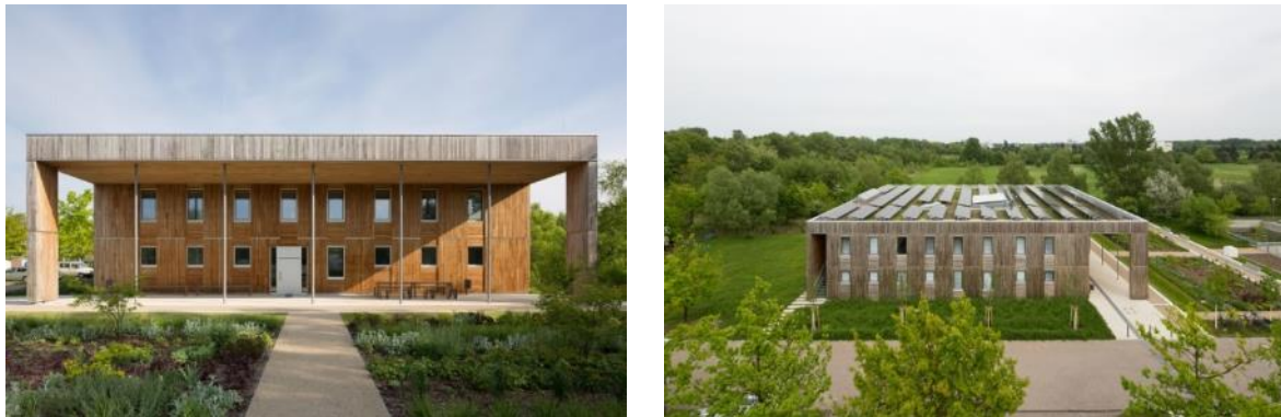
Figure 1: UBA 2019; view from south (left), view from west (right)
