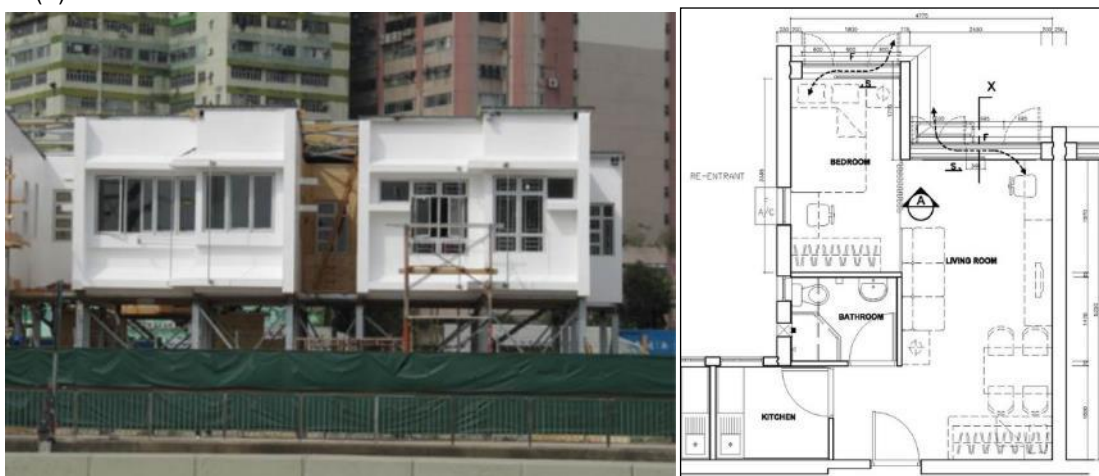
Figure 4: Mock-up flats for comparison of the performance of conventional window and acoustic window
