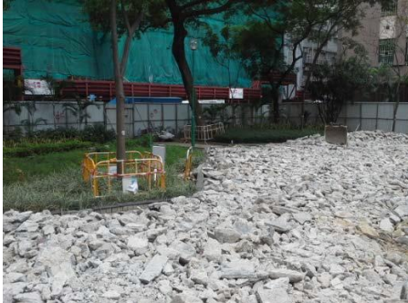
Demolished concrete was used in another site as filling materials
