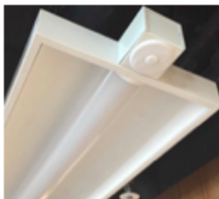
Occupancy sensors for lighting system
