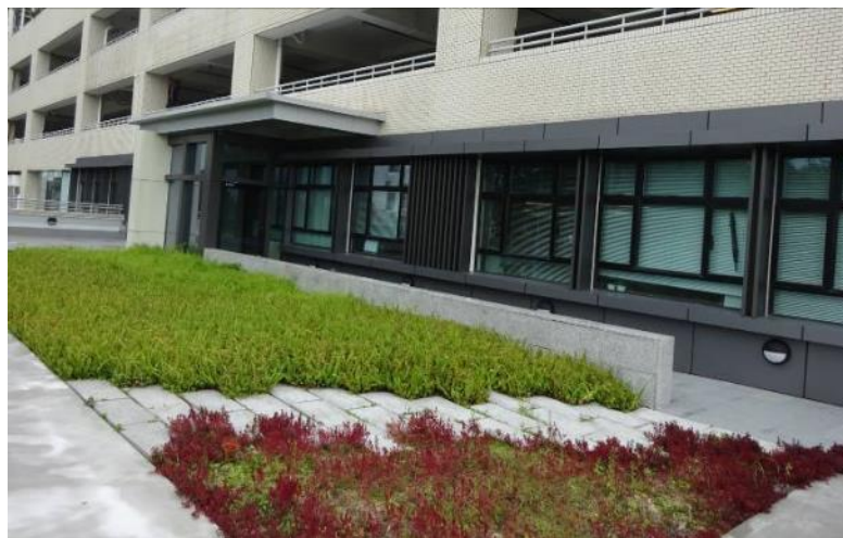
New green roof
