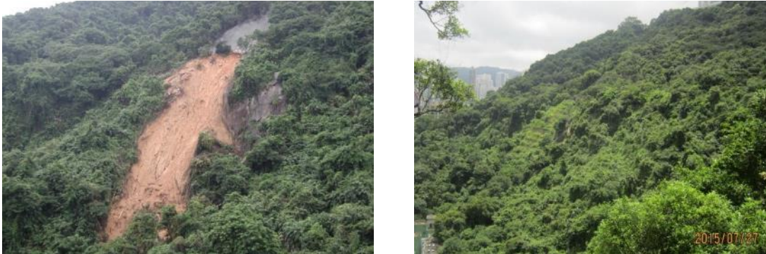
Figure 1: Slope greening above Bowen Road before (left photo) and after (right photo) works
