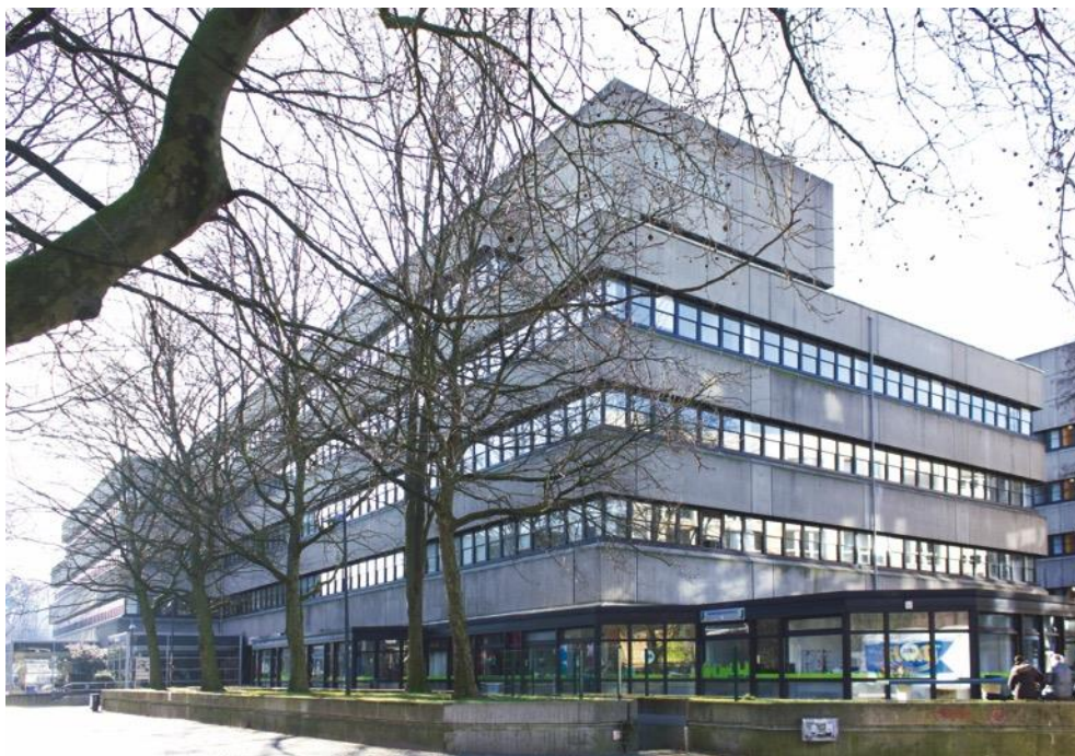
Figure 12: Photography of north façade corner, Von-Melle-Park 5, 2016. PASD Architekten. Feldmeier & Wrede. Photography taken by Maria Tumanovska, 02/2016.
