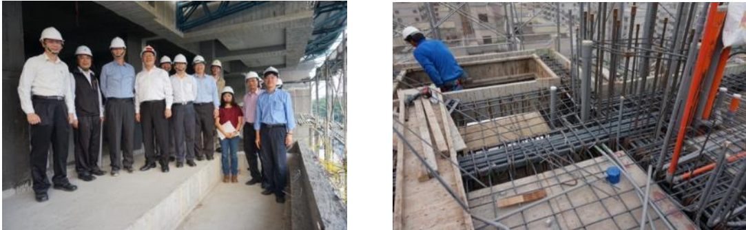
Figure 3: The field surveys on Kaohsiung house
