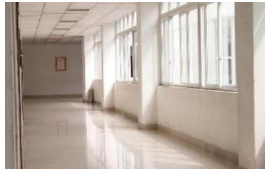
One-sided enclosed corridor school building (Type B)
